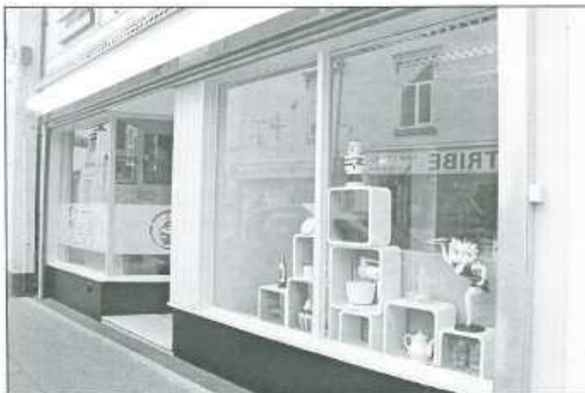
Crystals Cupcakes is a new shop in Dawley High Street and has used the grant to contribute towards the renovation works.
